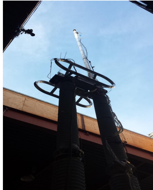
Figure 5, 500 kV SEECO switch, Mast Open
