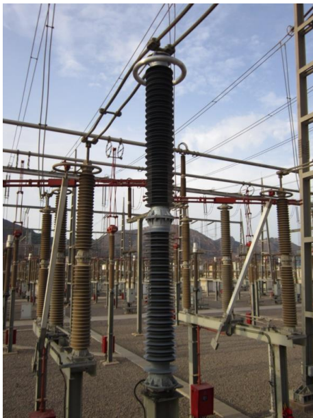
Fig. V: Replacement in 420kV AC substation with Hybrid solid core post insulators HC8 -1550
