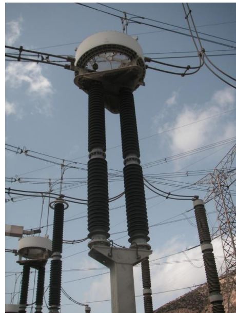
Fig. V: Replacement in 420kV AC substation with Hybrid solid core post insulators HC8 -1550
