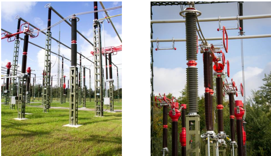
Fig. IV: Extension of 420kV AC substation with Hybrid solid core post insulators HC10 -1550 mod.
